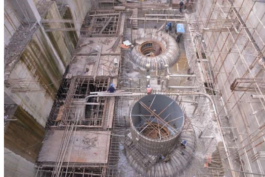
Figure 6 - Turbine Spiral Casing Installation
